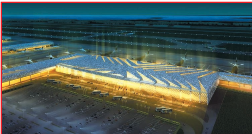
● A 'bird's eye' view of the terminal building
